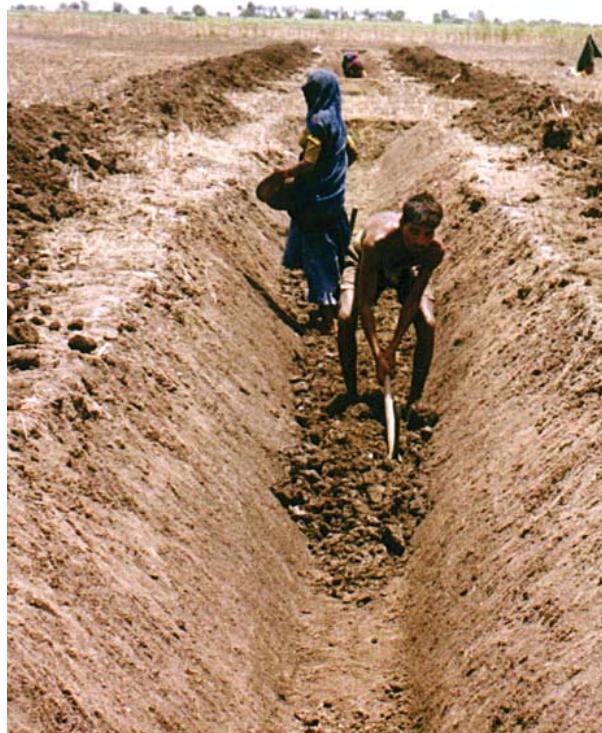
Manual installation of open drains
