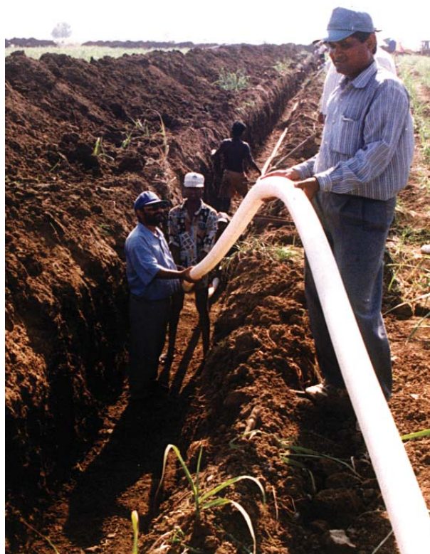
Manual installation of pipe drains
