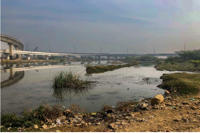
The Barapullah drain in New Delhi: one of the biggest open sewer systems
