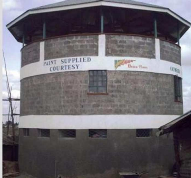
Anaerobic digester beneath the toilets;
